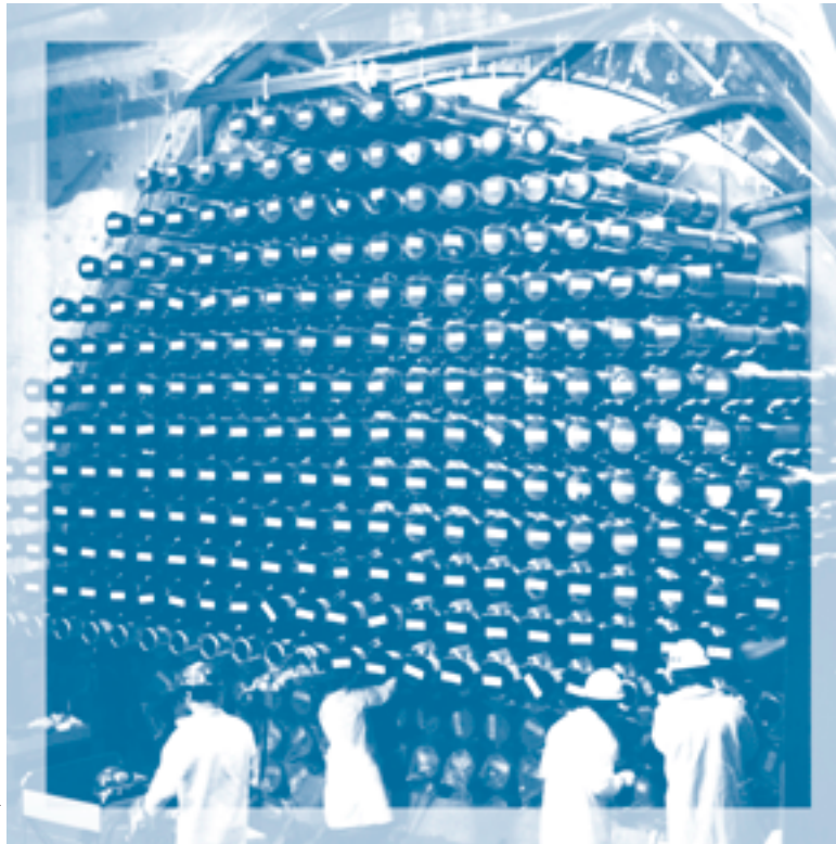
Installation of fuel rods at the Gentilly 2 nuclear power plant, Canada.
