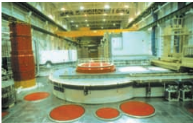
Inside the reactor hall of the Mochovce VVER unit in the Slovak Republic.
