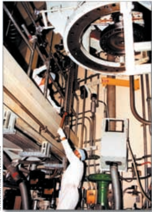
Reinstallation of the main reactor coolant pump after inspection and overhaul at the Beznau nuclear power plant, Switzerland.
