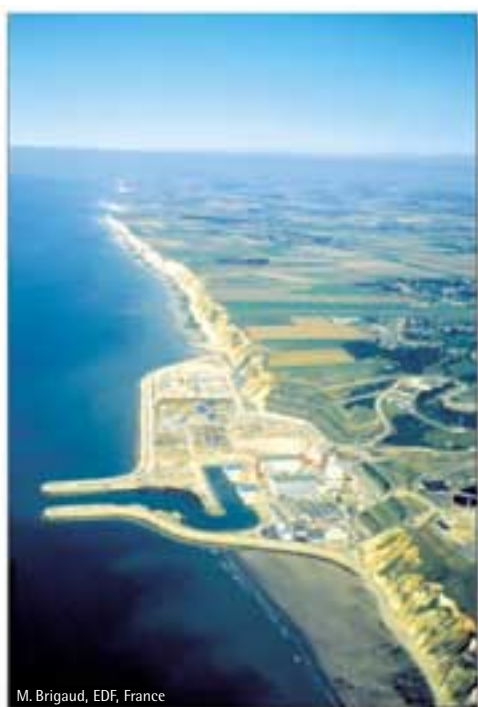
View of the Penly nuclear power plant, France.
