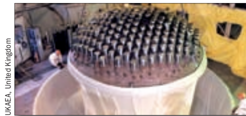
Decommissioning at Windscale, United Kingdom.
