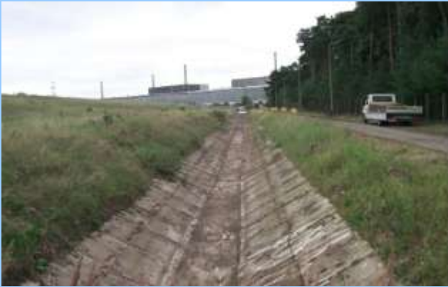
Discharge of radioactive substances during operation caused contamination
