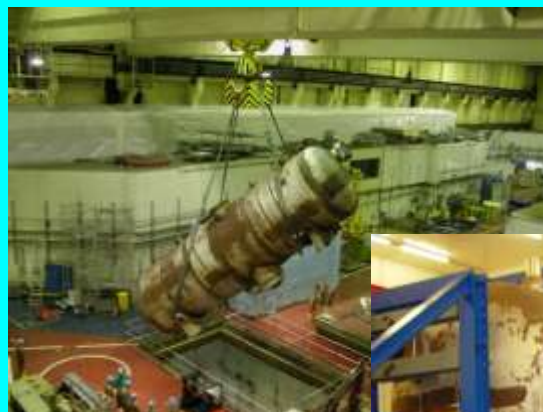
Removal and segmentation of a steam generator
