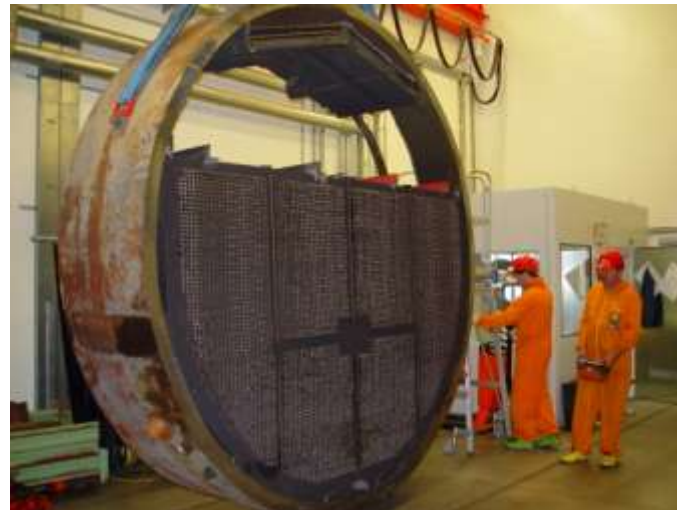
ISN Caisson 4: Segmentation of a steam generator
