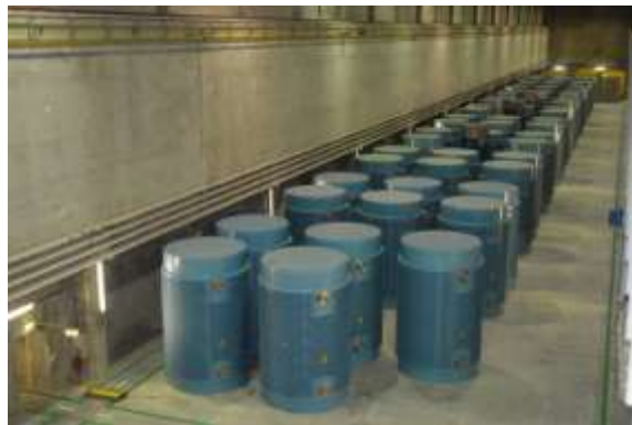
Hall 8 of the transport cask store in the ISN with 65 CASTOR casks
