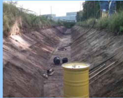
After removal of concrete slabs and cleaning
