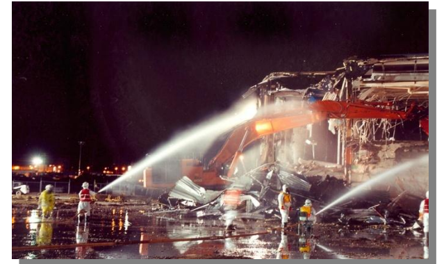
Nighttime demolition of a plutonium facility
