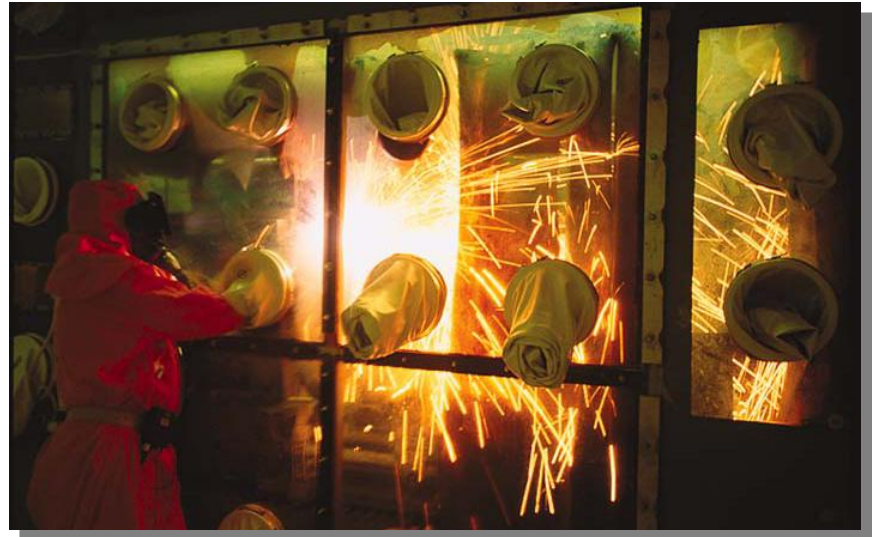
Cutting gloveboxes using plasma arc improved safety and productivity
