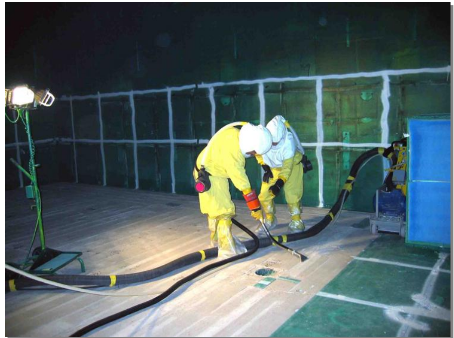
Workers decontaminate concrete flooring
