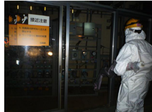
Reactor instrumentation rack
