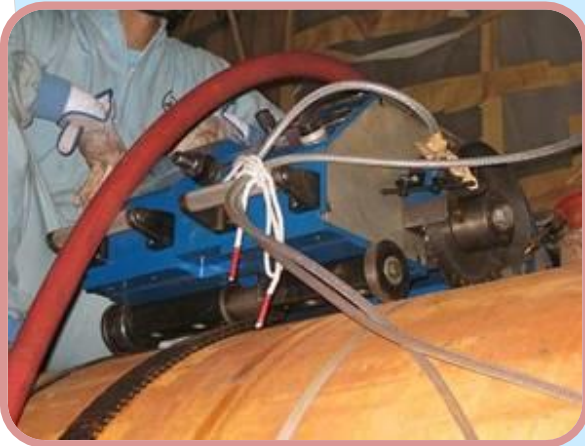
Orbital pipe cutting machine
