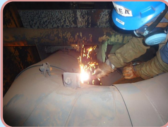
Cutting by a plasma cutting machine
