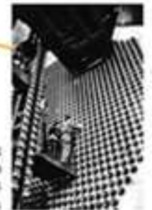
G1 (CEA, air cooled), 2 Mwe, 1956→ 1958 G2(CEA), 38 Mwe, 1958→ 1980 G3 (CEA), 38 Mwe, 1959→ 1984 +Chinon graphite sleeves stored in silos
