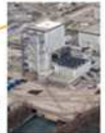
Bugey 1 (EDF) 540 MWe 1972→ 1994
