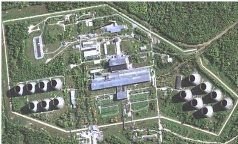
North site (area 11) – 2 industrial reactor plants
