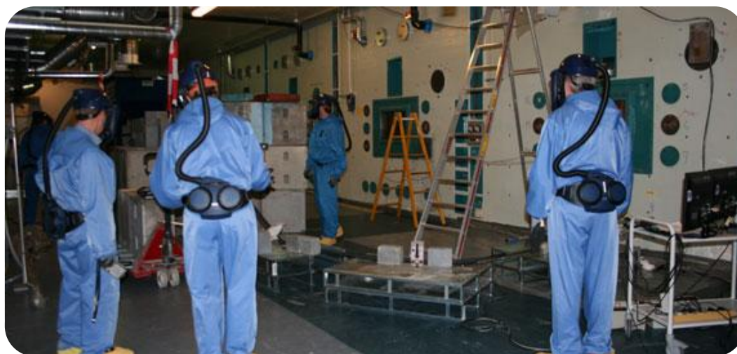
Figure 2, Preparation for removal of hot spots in the Hot Cell facility. The windows to the cells can be seen in the background.
