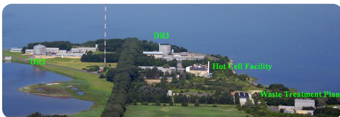
Figure 1, Overview image of the Risø peninsula and DD. The DR2 and the nuclear facilities DR3, Hot Cell and the Waste treatment plant are seen.
