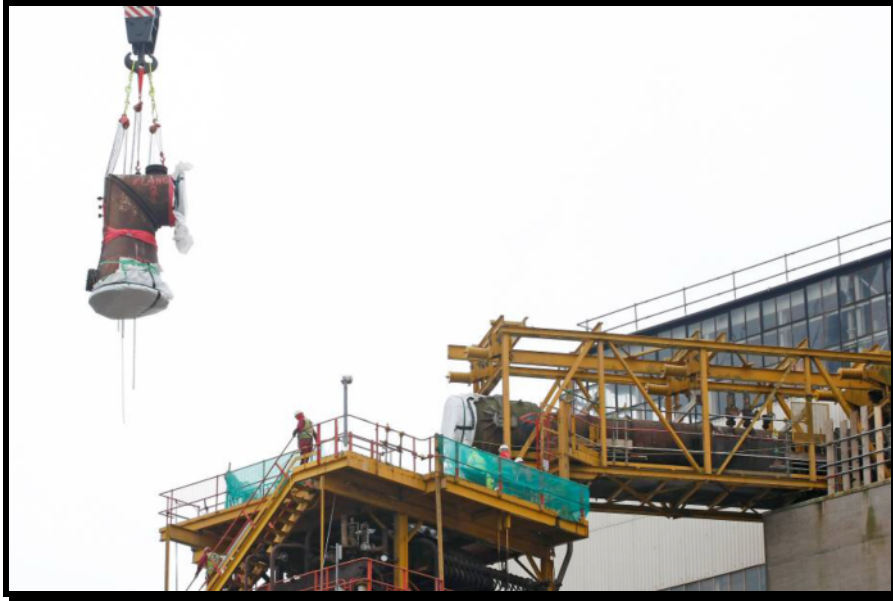
Picture 3. Top duct elbow being removed.
