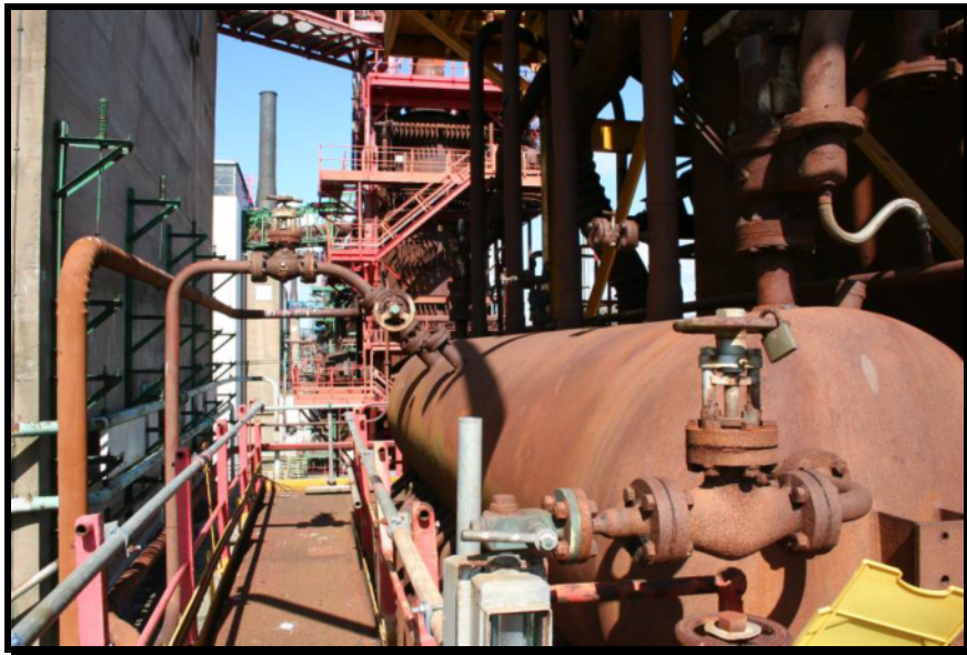
Picture 10. Example of a steam drum
