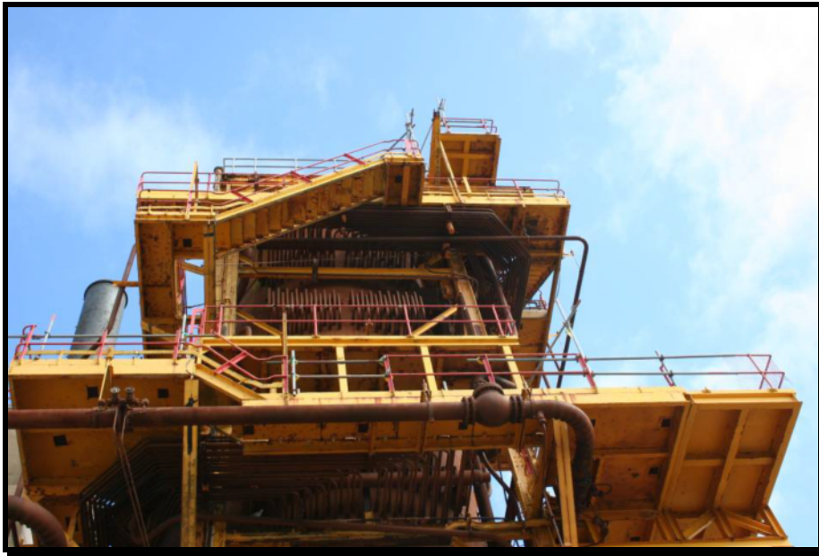
Picture 15. Upper level access platforms, gantries and stairways
