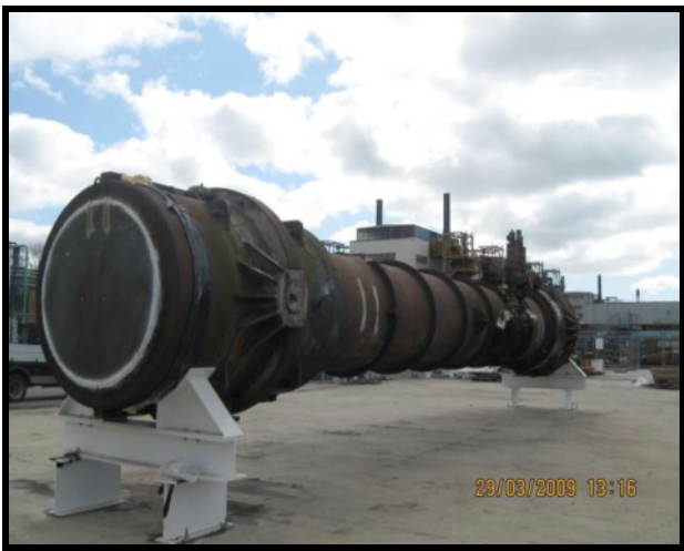
Picture 4. Top duct mid section removed from heat exchanger.
