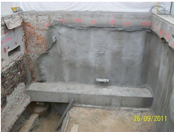
Fig. 8. Piling wall insulation
