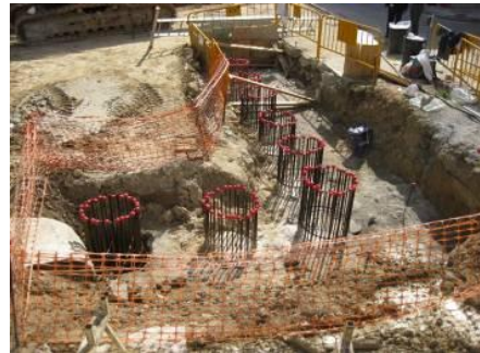
Fig.4: Construction of underground piling wall
