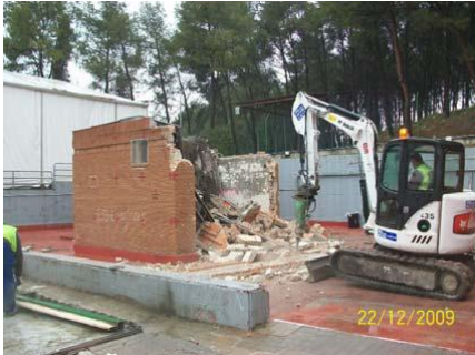
Fig. 3: Demolition of over structure
