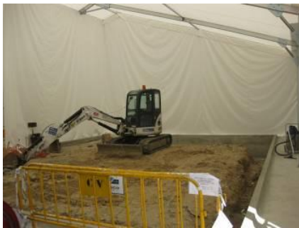
Fig.5: Soil excavation inside confinement tent
