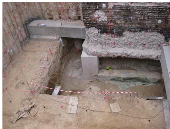
Fig. 7. Levels reached in the Lenteja excavation.
