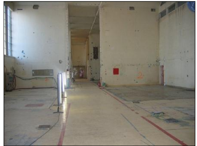
Before concrete decontamination
