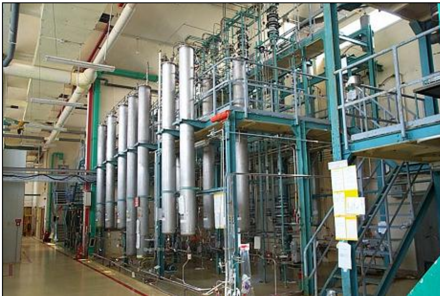
“Atelier D” before process equipment dismantling
