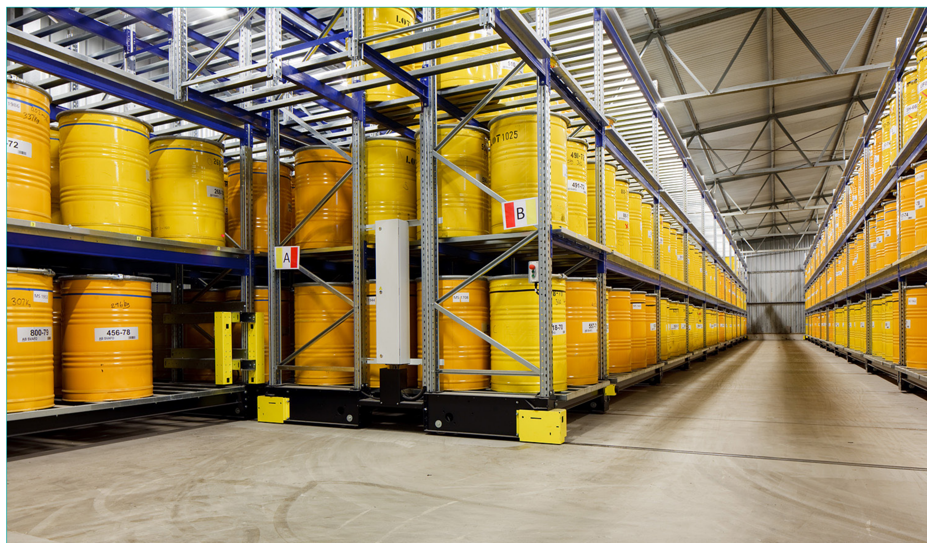
The AU building at Studsvik will become the interim storage facility for all characterised drums until their final disposal at the future SFL repository. An electrically controlled, racking system enabling access to each and every characterised drum is currently being installed as shown in the photo below.
