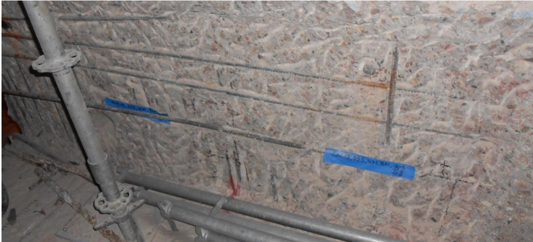
Figure 1: Reinforcement in a wall after removal of the outer concrete layer
