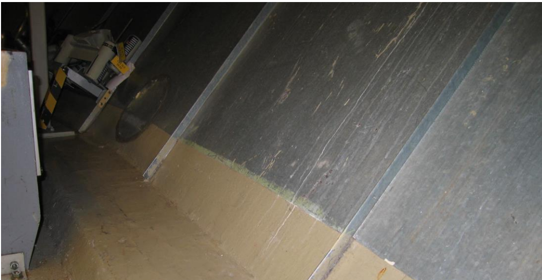
Figure 2: Metal cladding on concrete surfaces in a nuclear power plant
