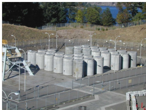
Loaded vertical storage systems at Trojan ISFSI
