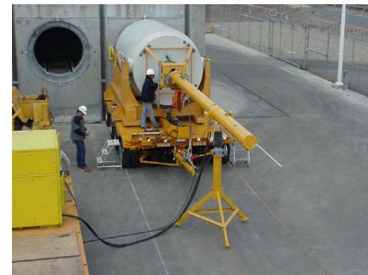
Transnuclear Horizontal Storage Module
