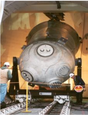
Figure 4 Removal of CY S/G Lower Assembly from the Containment Building
