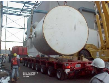
Figure 5 CY S/G Dome Lower on Transporter for Movement to Rail Spur
