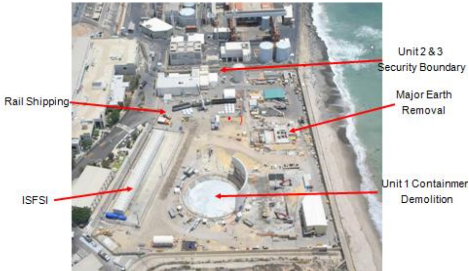
Figure 7 Concurrent Activities during the San Onofre Unit 1 Decommissioning
