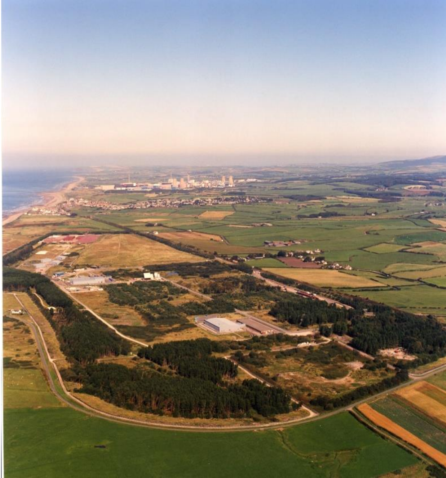
UK Low Level Waste Repository, Drigg, Cumbria
