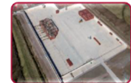
View of vault 9
