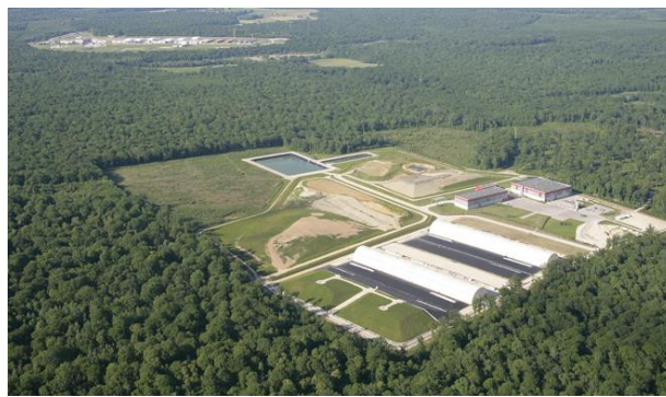
Fig. 2: Morvilliers disposal facility
