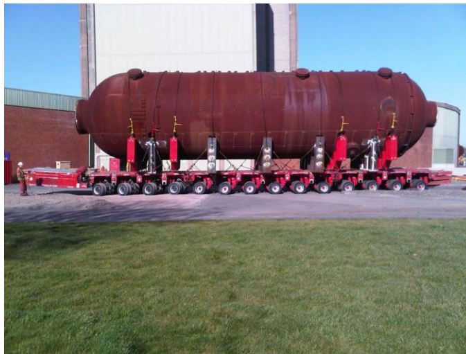
Figure 5 Photograph showing boiler loaded onto SPT
