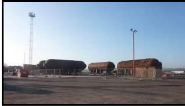
Figure 8 In-transit storage of boilers
