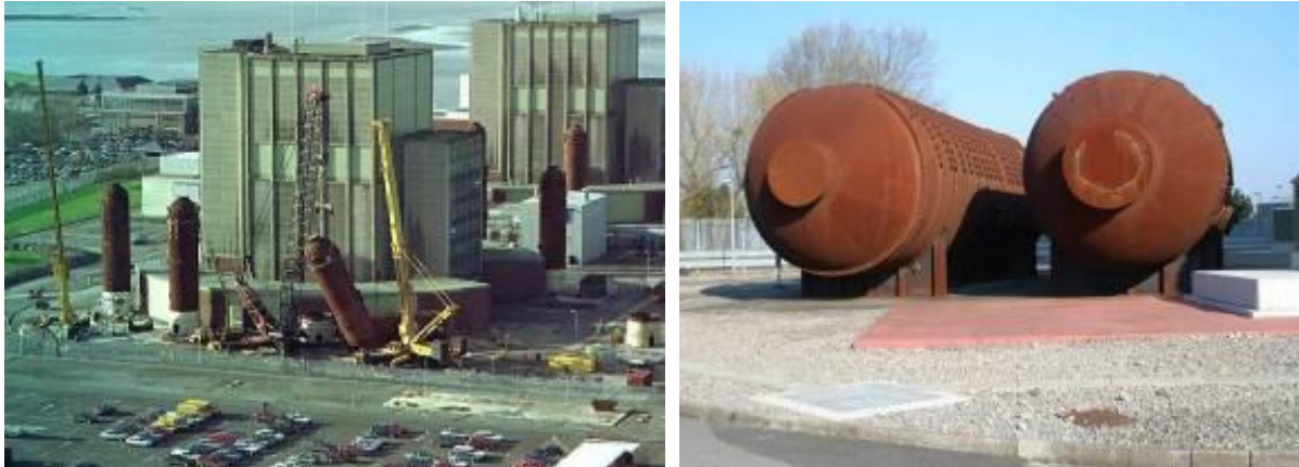
Figure 3 Photographs showing boiler lowering and final example of one storage location
